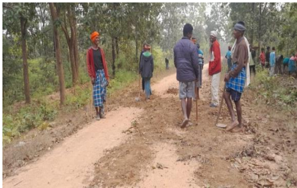
Road repairing by villagers at picnic spot
